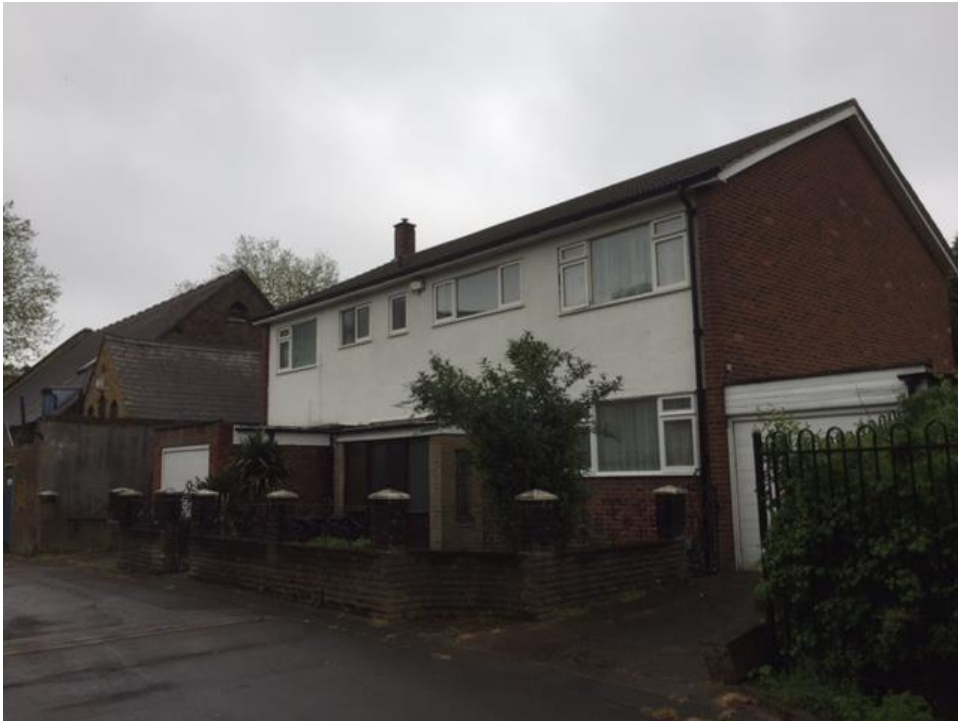
Image 2: Front elevation of 38 Hilldrop Lane taken from north
